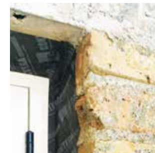
Thermal bridge free window installation with PHONOTHERM 200
