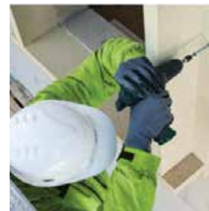
Thermal bridge free window installation with PHONOTHERM 200
