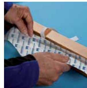
Thermal bridge free window installation with PHONOTHERM 200
