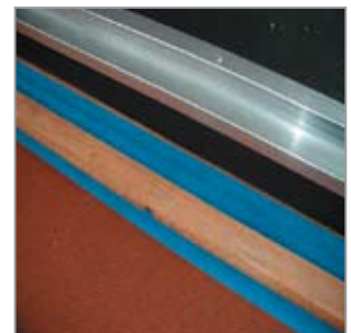
Skylight window Make connection using BUDAX TOP 75mm or 150mm, depending on requirements.
