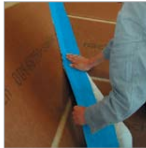
Channels and ridges Use BUDAX TOP in 150 mm for sealing channels and ridges.
