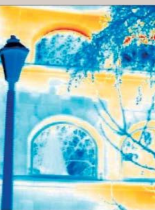
Infrared image of the Herrenschießhaus
