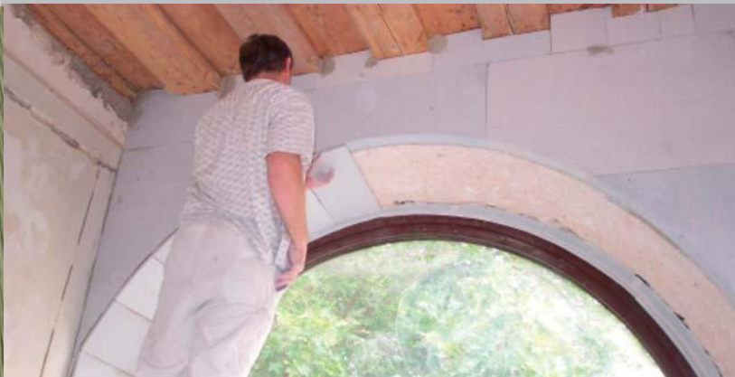
Arch with soffit panels
