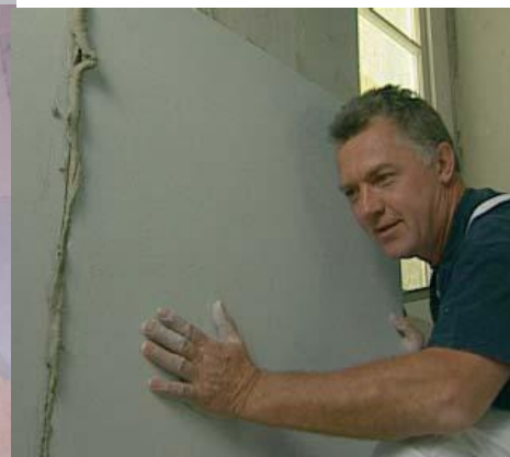
Positioning and pressing the panels into place
