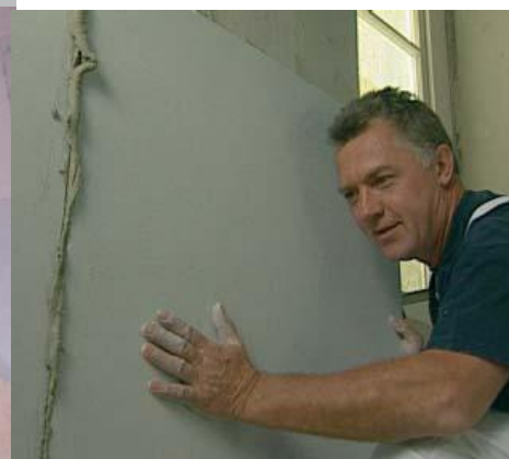
Positioning and pressing the panels into place
