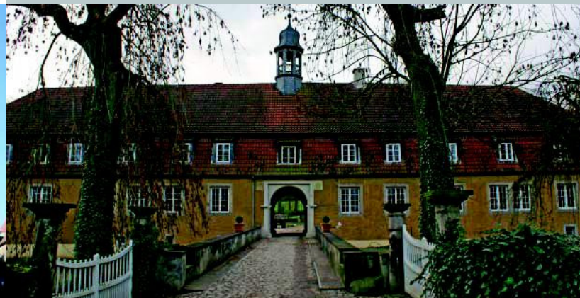
Residential building in Kirchlengern
