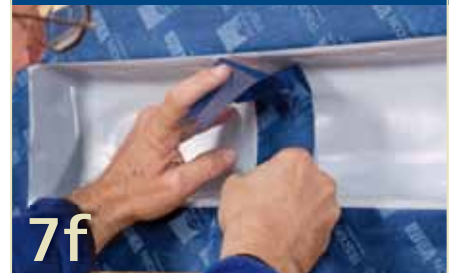
Enlarging: Taping over the overlaps
