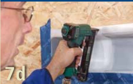
Enlarging: Fixing the overlap
