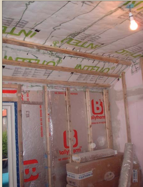
(left) Friction fit hemp wool insulation in the services zone; (below) dry-lining and air-tightness measures to improve the existing house
