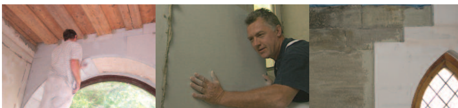
Figure 2 (below): Thermally upgrading a building internally with Calsitherm Climate Board
