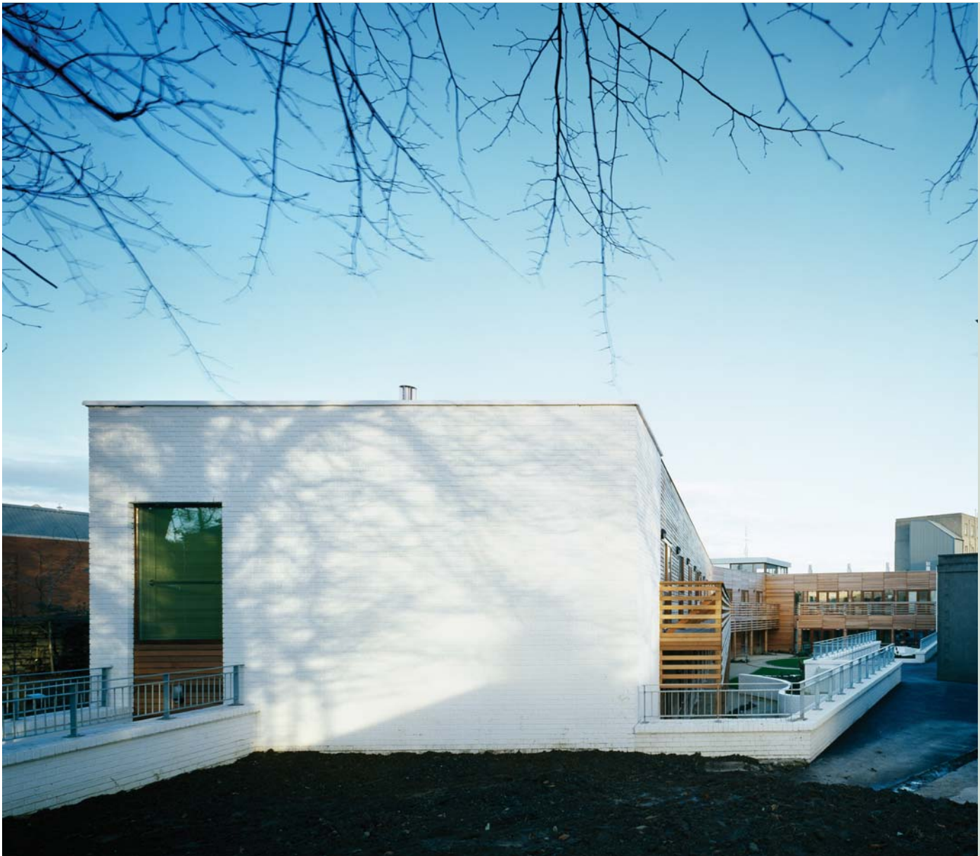
(above) The north walls onto the North Circular Road are heavily insulated cavity walls with a U-value of 0.19 W/m 2 K with a brick outerleaf painted with white Beekosil mineral paint.
