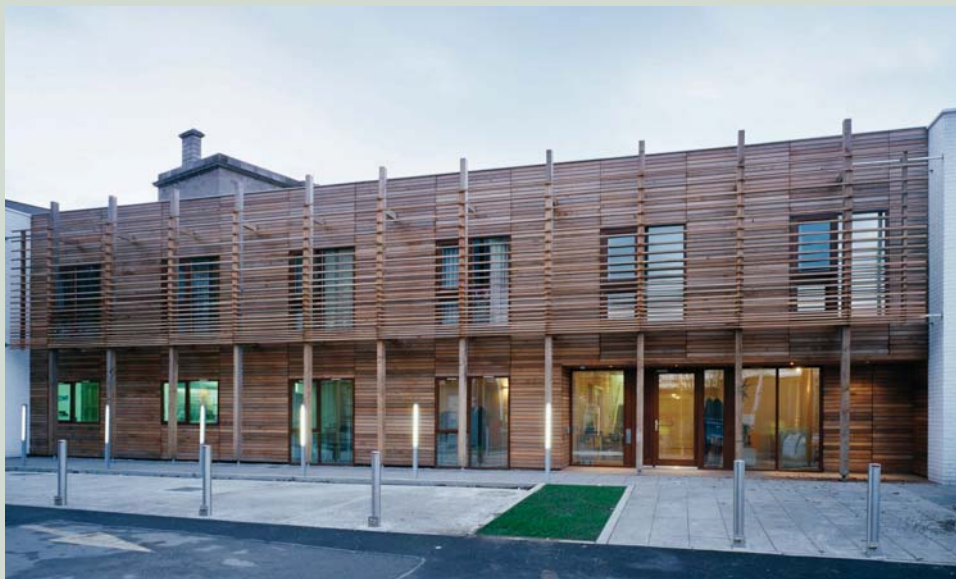
The building is a hybrid of masonry and timber framed construction in order to achieve a balance between effective insulation and thermal mass. The wall onto the forecourt to the east (above) and the garden court to the south (below) contrasts with the solidity and weight of the masonry walls (top). These walls are heavily insulated timber framed and clad walls with a U-value of 0.17 W/m 2 K.
