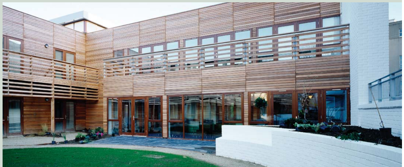
The building is a hybrid of masonry and timber framed construction in order to achieve a balance between effective insulation and thermal mass. The wall onto the forecourt to the east (above) and the garden court to the south (below) contrasts with the solidity and weight of the masonry walls (top). These walls are heavily insulated timber framed and clad walls with a U-value of 0.17 W/m 2 K.
