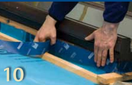
Detail: Rooflight window
