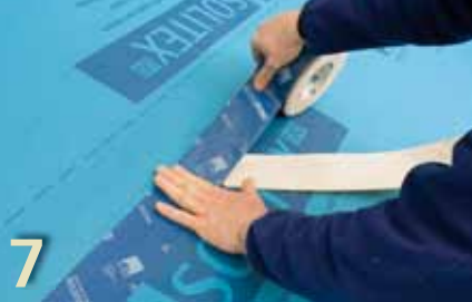
Joining SOLITEX roof underlay
