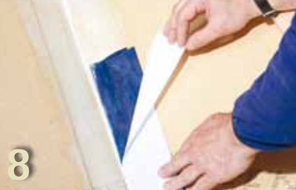
Joining softwood fibre roof underlay
