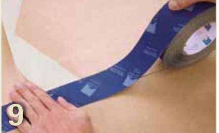
Joining wood fibre boards
