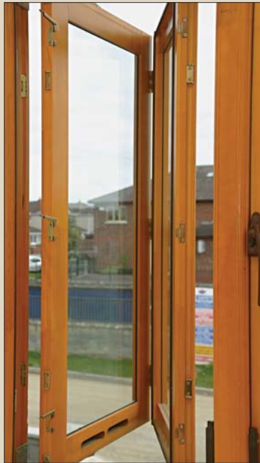
The supply air windows (above) open here to reveal their innovative yet low-tech workings, are made with two single glazed sashes with a 30 mm gap between the panes of glass
