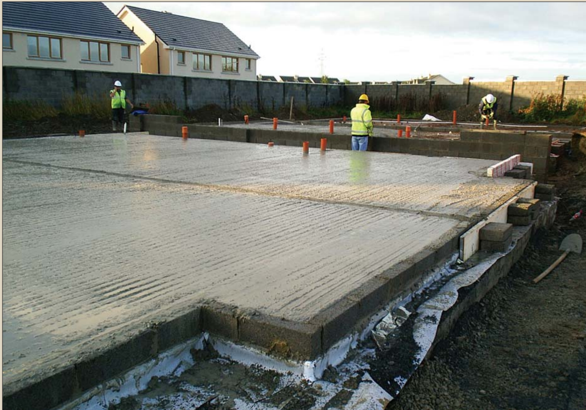
(clockwise from above) The Ecocem ground granulated blast slag based slab prior to a power float finish; achieving the highest possible airtightness levels is key to the performance of the homes at Easton Mews, as seen here in this detail to the plastered block reveal; an airtight membrane to a party wall at first floor level; a plasterboard reveal covering airtight detail; and an airtight membrane under joist hangers
