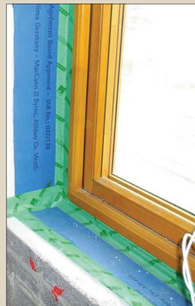
(clockwise from above) The Ecocem ground granulated blast slag based slab prior to a power float finish; achieving the highest possible airtightness levels is key to the performance of the homes at Easton Mews, as seen here in this detail to the plastered block reveal; an airtight membrane to a party wall at first floor level; a plasterboard reveal covering airtight detail; and an airtight membrane under joist hangers
