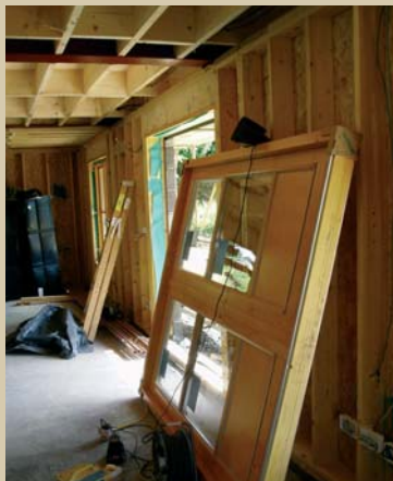
(anti clockwise from bottom left): the pre-engineered timber frame structure takes shape with walls, roof and doors being erected
