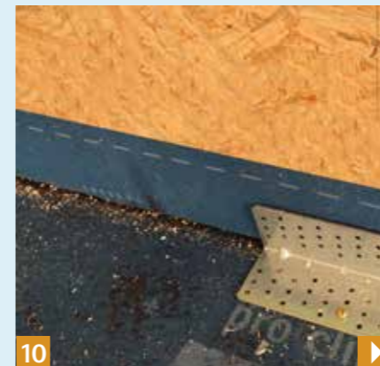
10 Fold wall joints up by about 10 – 15 cm above the horizontal surface.
