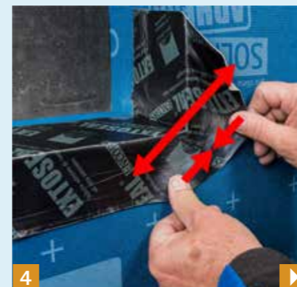
4 Form the sub-sill flashing using EXTOSEAL ENCORS.
