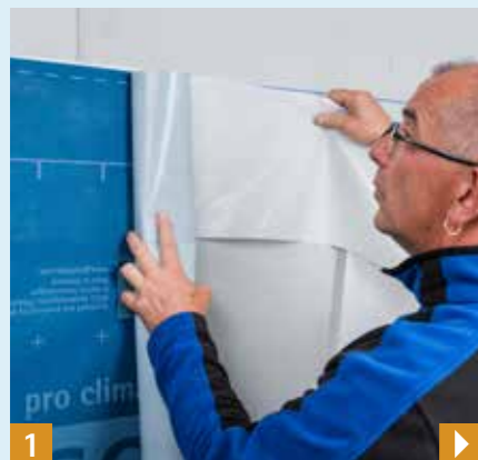
1 The membranes are generally installed horizontally.
