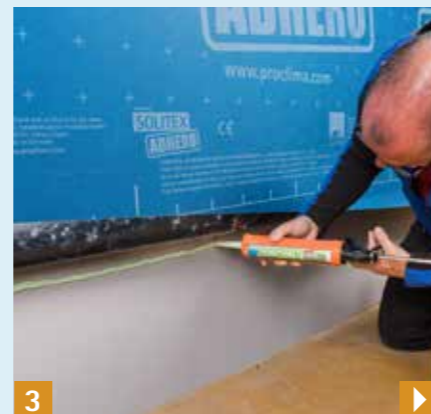
3 Sealing to rough subsurfaces using ORCON F.
