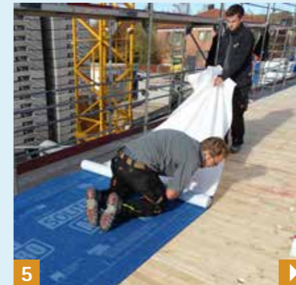
5 ... and gradually stick it to the subsurface.
