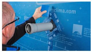
**22. Pipe feed-throughs with ROFLEX** Seal pipe feed-throughs with a suitable ROFLEX grommet. Stick the grommet to the subsurface using TESCON VANA. Rub over the stuck surface using PRESSFIX XL
