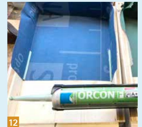
12 Additionally seal membrane overlaps at protruding walls using ORCON F.
