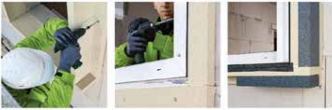
Thermal bridge free window installation with PHONOTHERM 200
