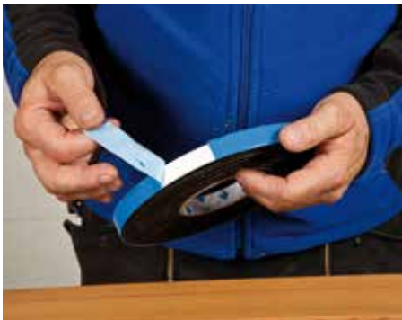
Cut the outer protective film with a utility knife and remove this film.
