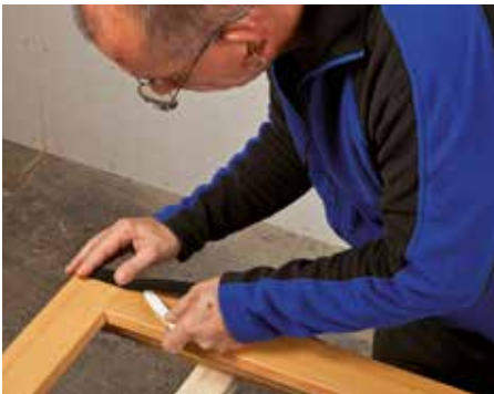
Remove the release film, align the tape straight on the frame and gradually stick it in place. The tape must not be visible after installation (allow a recess of approx. 1-2 mm; 1/16").
