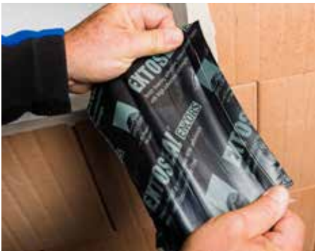
Very elastic – adapts flexibly to subsurfaces and corners.
