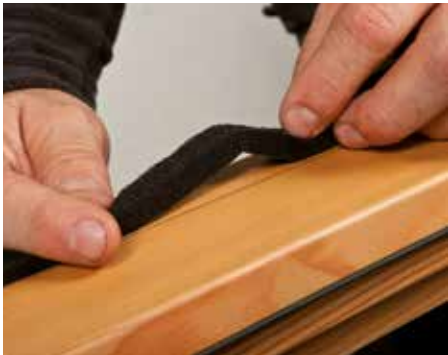
Allow for a small amount of slack in the tape when sticking it in place, particularly near joints – do not stretch the tape!
