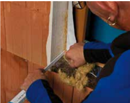
Install the window and insulate the joint
