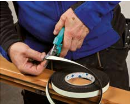
Roll off a length of CONTEGA FIDEN EXO and cut off the overcompressed start of the tape (approx. 2 cm; 3/4").
