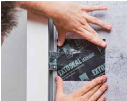
Waterproof taping of angle brackets.
