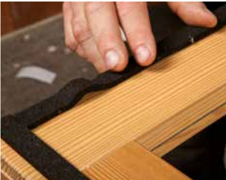
Stick the tape all around the window frame. Use a separate length of CONTEGA FIDEN EXO on each side, and use butt-joints at the corners. Allow for a small amount of slack near the corners.
