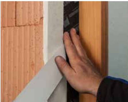
Stick CONTEGA SOLIDO EXO-D onto the reveal and rub into place
