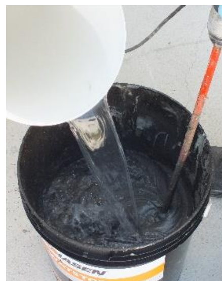
Figure 21: Add clean water to the mix to dilute the mixture until the optimum consistency is reached according to the type of application envisaged by the project.
