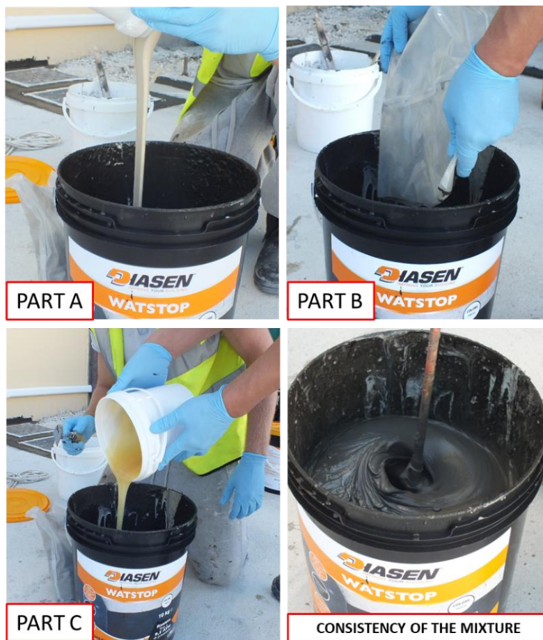
Figure 20: Steps in the preparation of the tricomponent mixture - WATstop
