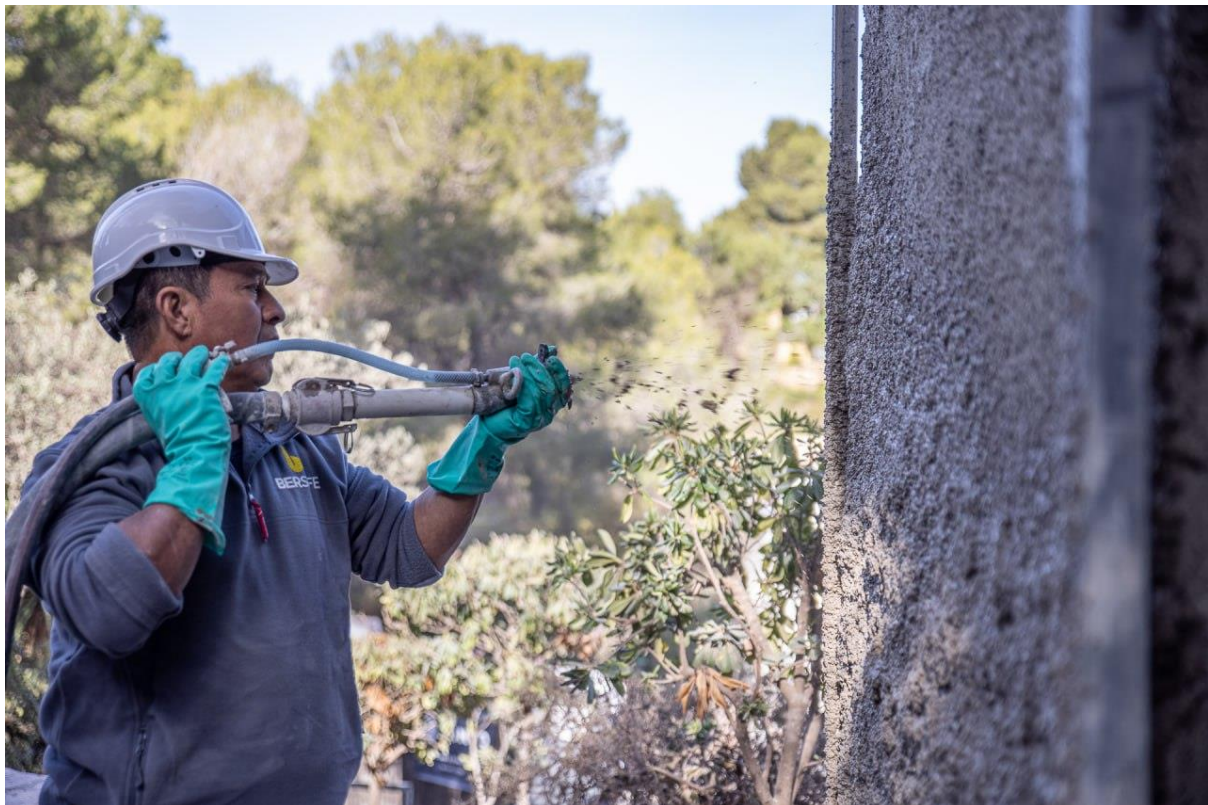
Figure 16: Application of Diathonite Evolution premixed plaster on brick and stone substrates by plastering machine
