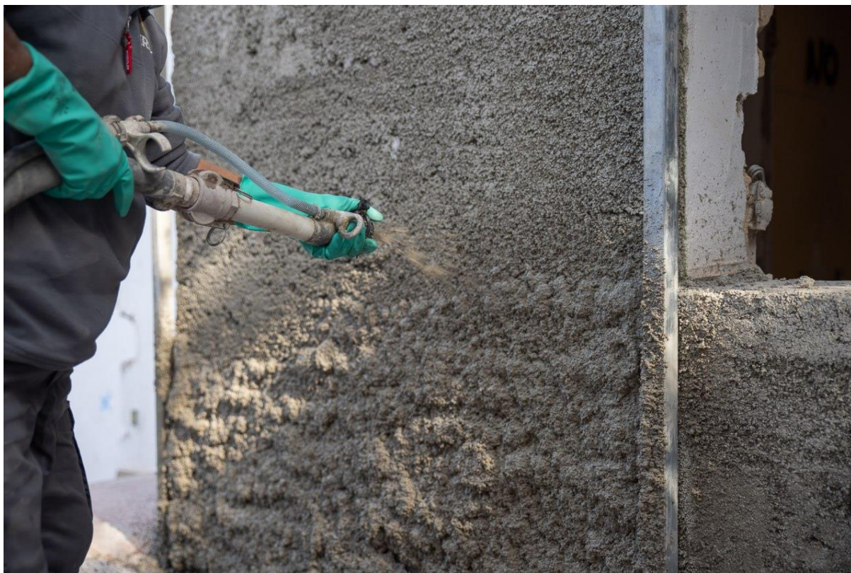
Figure 17: Application of Diathonite Evolution premixed plaster on brick and stone substrates by plastering machine
