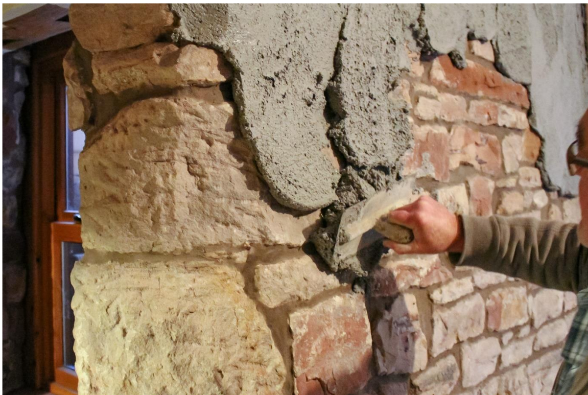
Figure 11: The cork-based premixed lightweight plaster for thermal insulation Diathonite Evolution, applied by hand with trowel/ trowel
