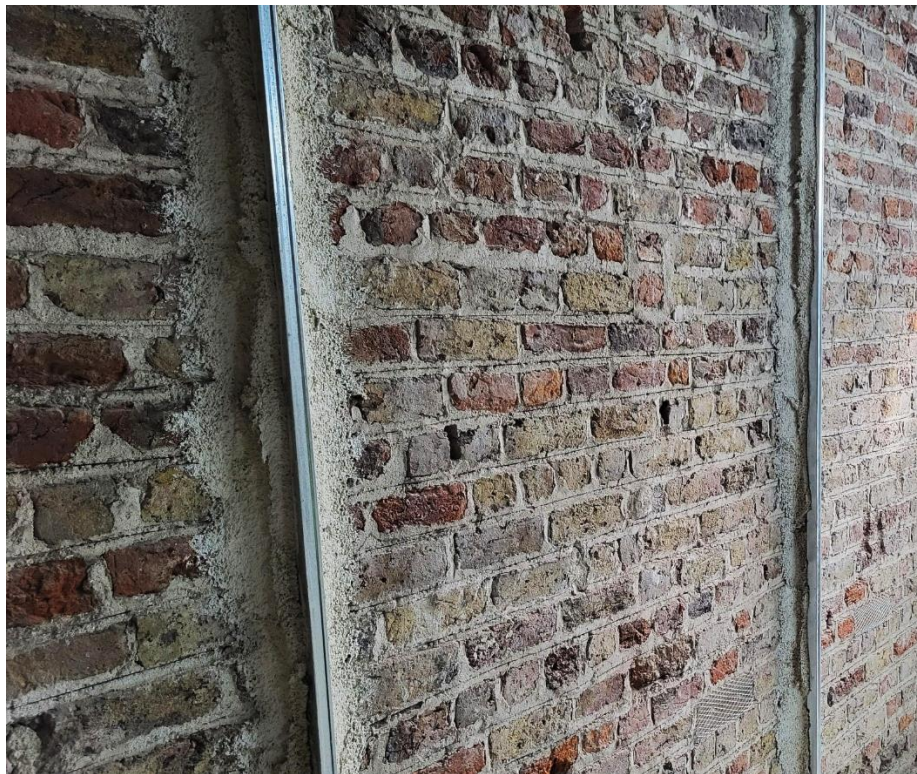
Figure 9: Aluminium battens or gauges embedded within plaster on the wall used as reference points when laying plaster
