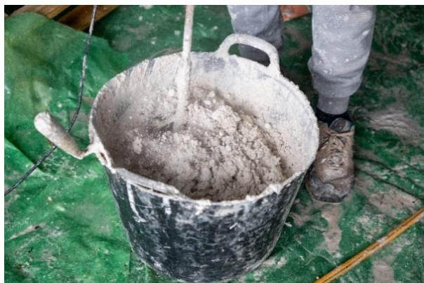
Figure 7: Image of drill mixer mixing Diathonite Evolution thermal plaster
