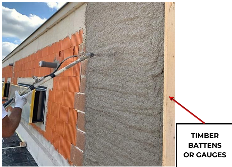
Figure 10: Practical example of wooden battens embedded within plaster vertically on a wall, used as reference points during the application of Diathonite Evolution plaster with plastering machine
