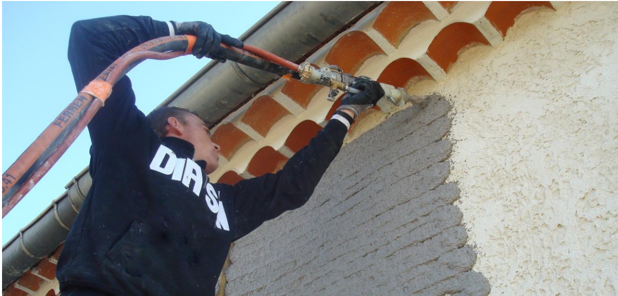
Figure 8: the cork-based premixed lightweight plaster for thermal insulation Diathonite Evolution applied with spray plastering machine
