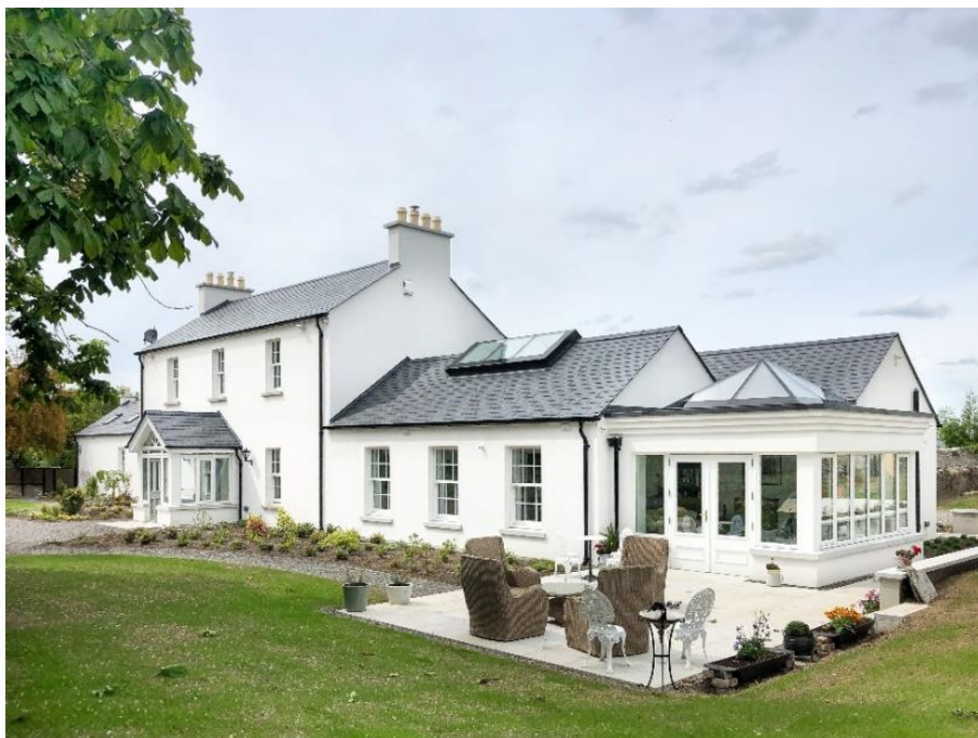
Figure 18: Smooth Argatherm finish over Diathonite Evolution (project: Clane Retrofit , Co. Kildare)
