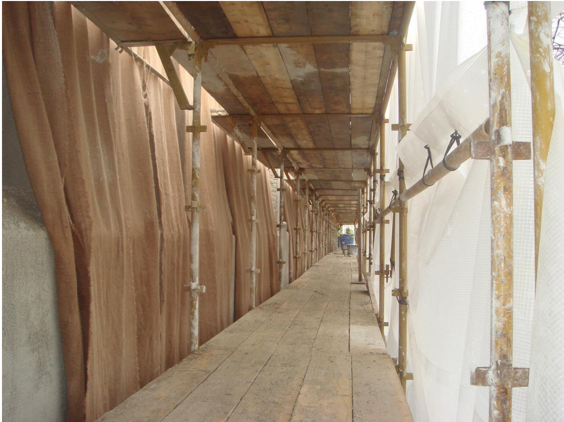
Figure 30: Robust weather protection of façade with scaffold, hessian and weathertight tarpaulin outside. Project – Peach House, Aras an Uachtarain, Dublin, Ireland
