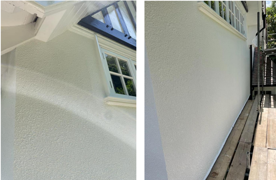
Figure 19: Argatherm with "dash effect" over Diathonite Evolution (images provided by Eco-Renovation UK)
