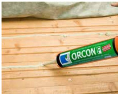
... for vapour checks underneath external roof insulation,
