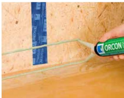
... and floor joints with wood-based panels,
