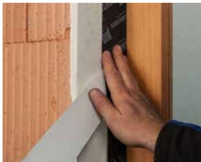
Stick CONTEGA SOLIDO EXO-D onto the reveal and rub into place
