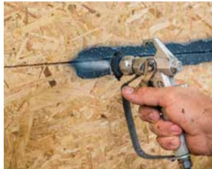
... joints between wood-based panels,
