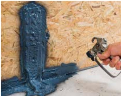
Airtight spraying over angle brackets,
