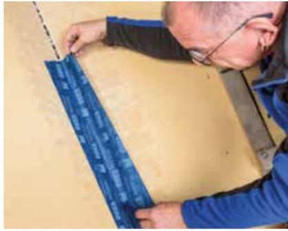
Tapes can be stuck directly onto recently applied primer.
