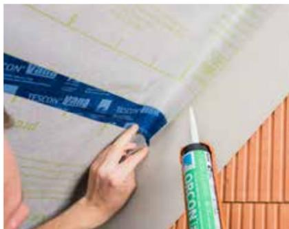
Joint adhesive for interior airtightness membranes,
