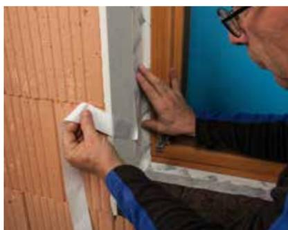
Stick onto the reveal and rub into place
