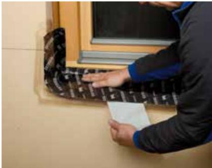
Can be used to create sub-sill flashing.
