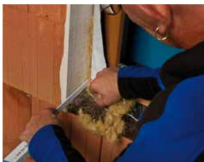
Install the window and insulate the joint
