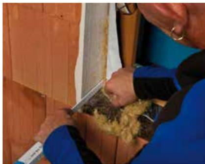
Install the window and insulate the joint
