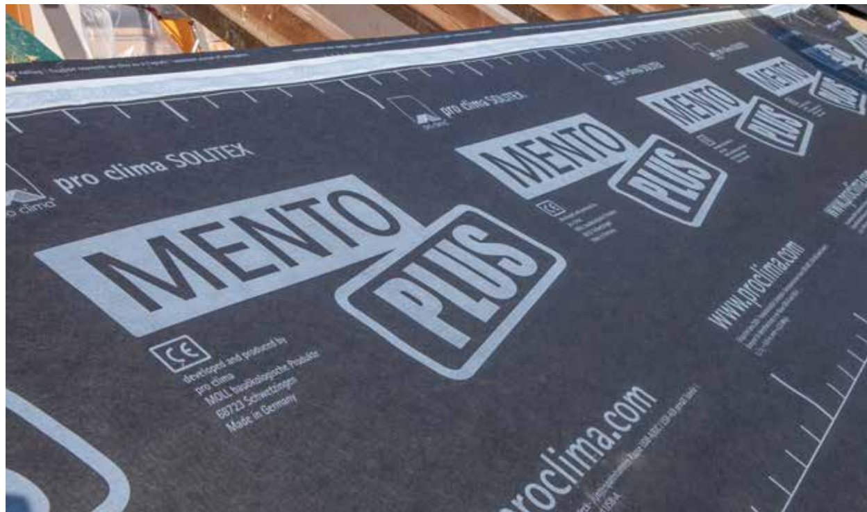
The roofing underlay membranes in the SOLITEX MENTO series have high resistance to ageing and are extremely watertight, but are diffusion-open. Their monolithic SOLITEX functional film provides ideal protection on the outside for the insulation.
