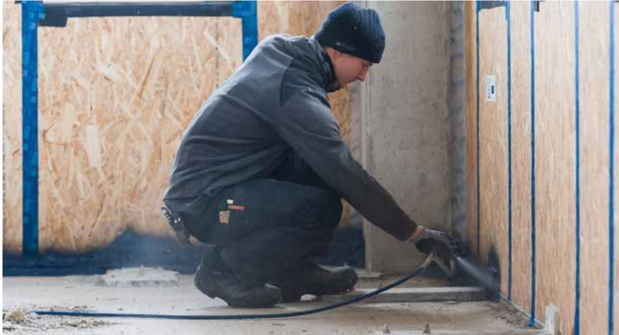
Our spray-on sealant saves a lot of labour time on site and is very versatile, particularly for challenging connections.
